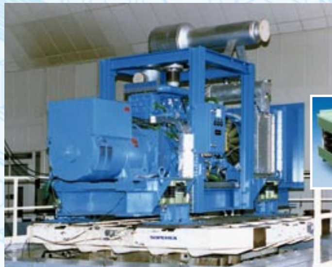
Vibration insulation with helical springs Source: www.gerb.com
