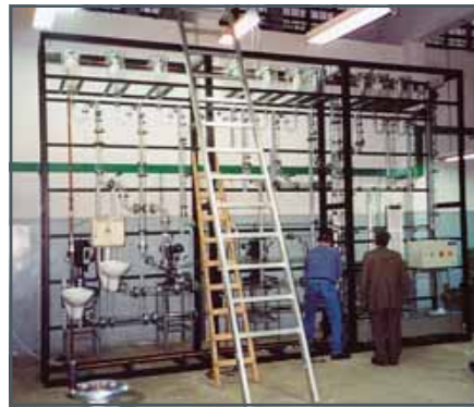
Installation of system at customer's site
